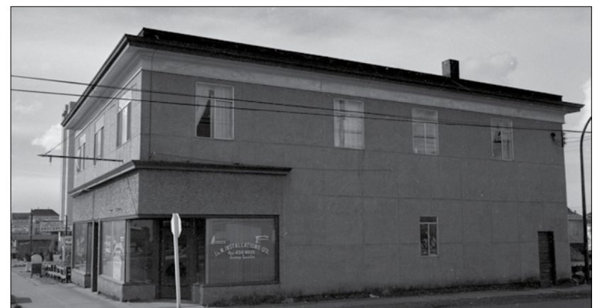
5103 Joyce and Vanness, on the SW corner. Photo taken in 1974. Vancouver Archives, CVA 786-98.13
