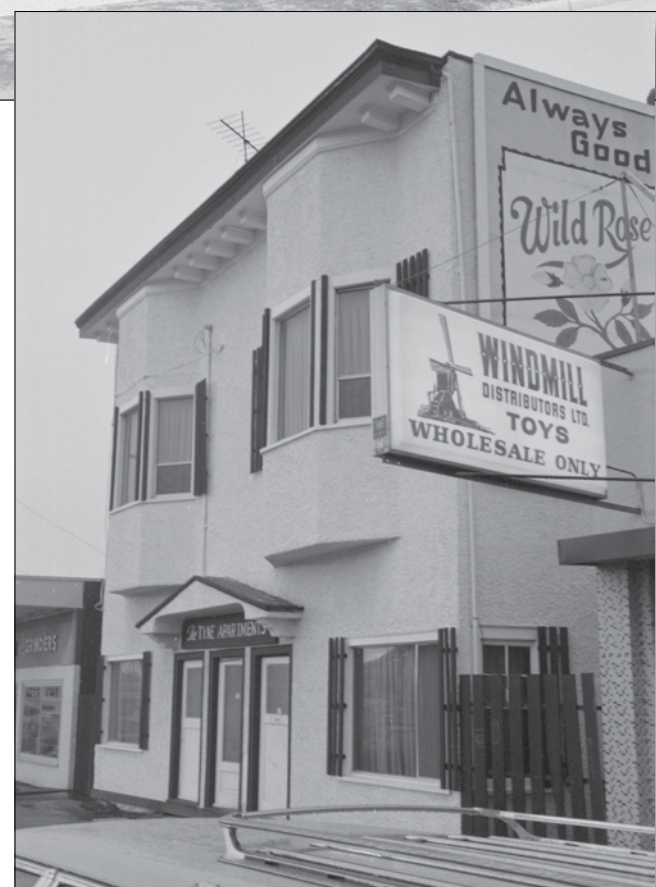
Tyne Apartments. Vancouver Archives photo, 1978; CVA 1093-04480.
